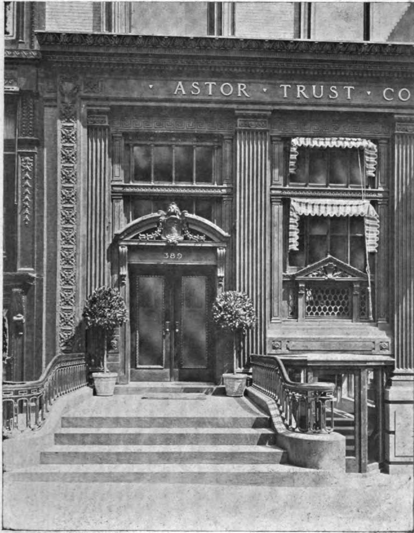
MAIN ENTRANCE, FIFTH AVENUE.
